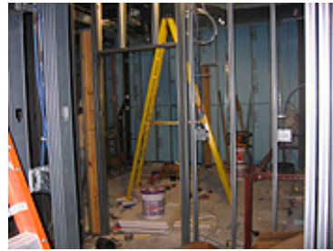
First floor office in Admissions is framed out.
