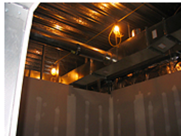
Second floor office reading for drop ceiling lighting and tile installation.
