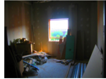
4th floor office, looking south toward Chestnut Street.
