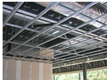
Second floor office reading for drop ceiling lighting and tile installation.
