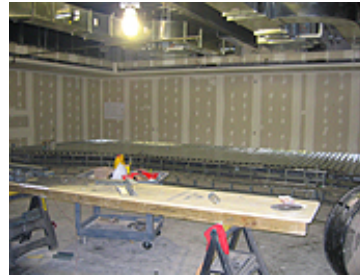
2nd floor: moot courtroom overflow area undergoes drywall installation and spackling.
