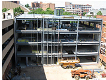
5.24.06: Aluminum studs being erected for outer wall.
