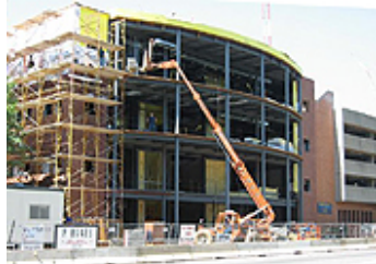
6.15.06: Laying of the brick on front and sides of building.
