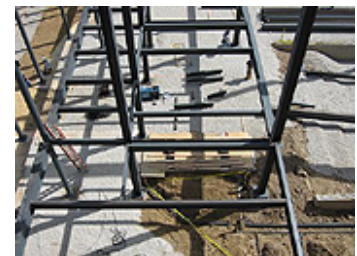
04.03.06: Steel cross-beams for second floor begun.
