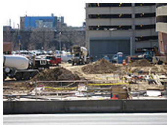
3.20.06: Pouring the concrete foundation.
