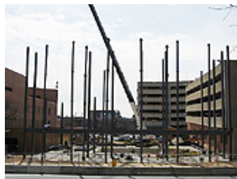
3.27.06: The steel has arrived!
