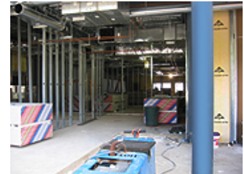
7.31.06: View inside atrium/lobby area; adding the interior drywall.
