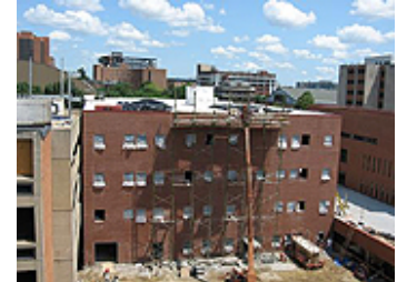
6.29.06: Rear of building brickwork is finished.
