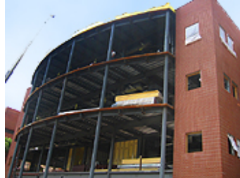
6.22.06: Close-up of atrium and finished brickwork.
