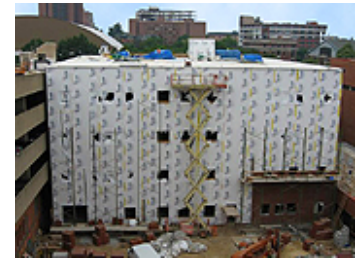
6.05.06: Insulation is applied to rear exterior.
