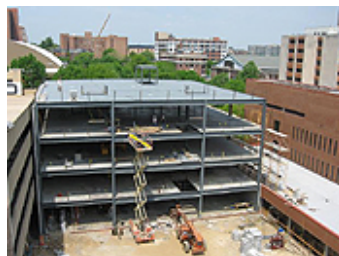
5.08.06: Rear view of building with all four floors framed out.
