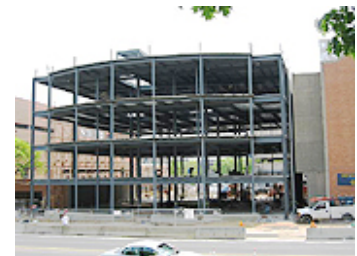
5.15.06: Front view of building with bowed window/2-storey atrium.
