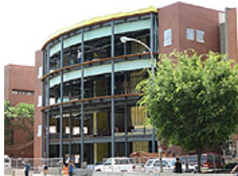
7.10.06: Preparations underway for adding the interior drywall.
