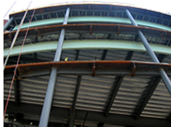
7.24.06: Close-up of atrium. Glass will be installed on all four floors.
