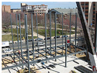
04.10.06: Crane adds more steel; seen from the rear of the building.
